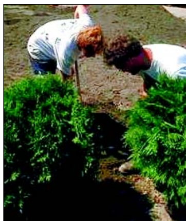
Don't go digging before you know where your lines are located.
